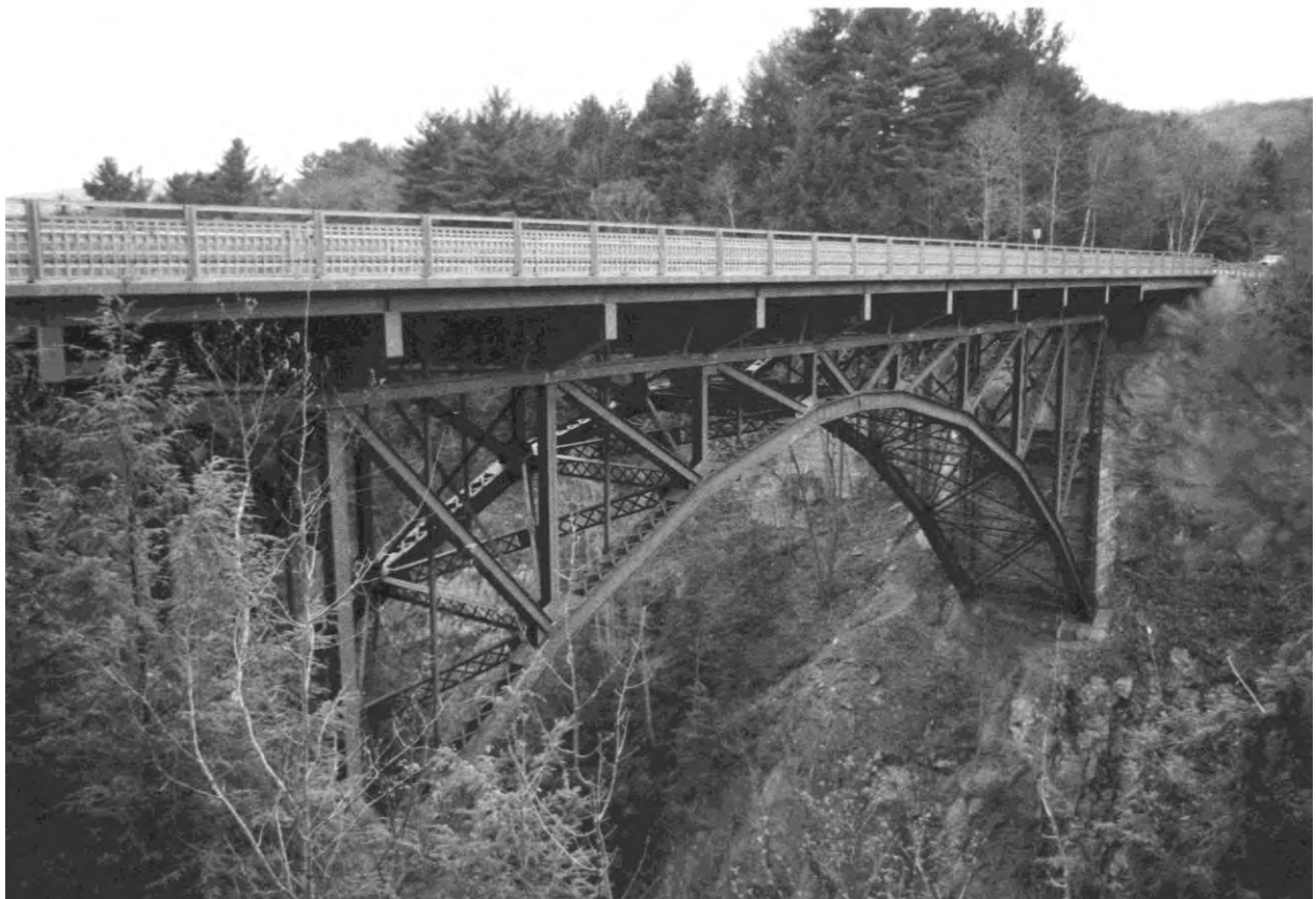
Figure 5. Quechee Gorge Bridge looking northeast. Image from 1990 NRHP nomination. Note contemporary rails.
