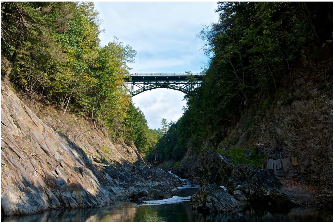
Figure 1. Quechee Gorge Bridge (Bridge No. 61), looking south
