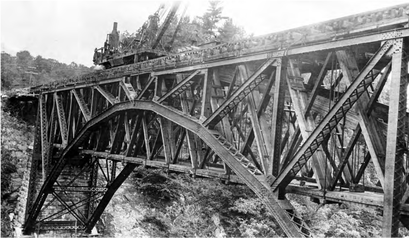
Figure 2. Construction of Quechee Gorge Bridge in 1911.
