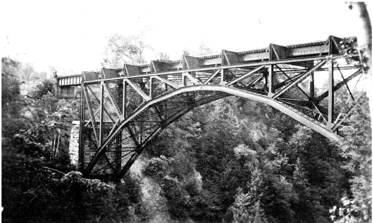
Figure 3. Completed bridge in 1911. Note rail deck.
