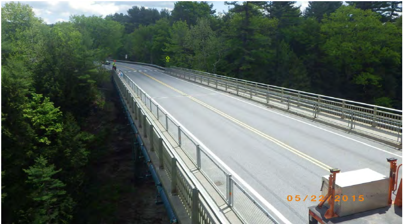
Figure 6. Contemporary rails on the Quechee Gorge Bridge, looking west.
