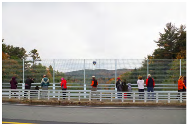
Temporary Wire Mesh Alternative:
