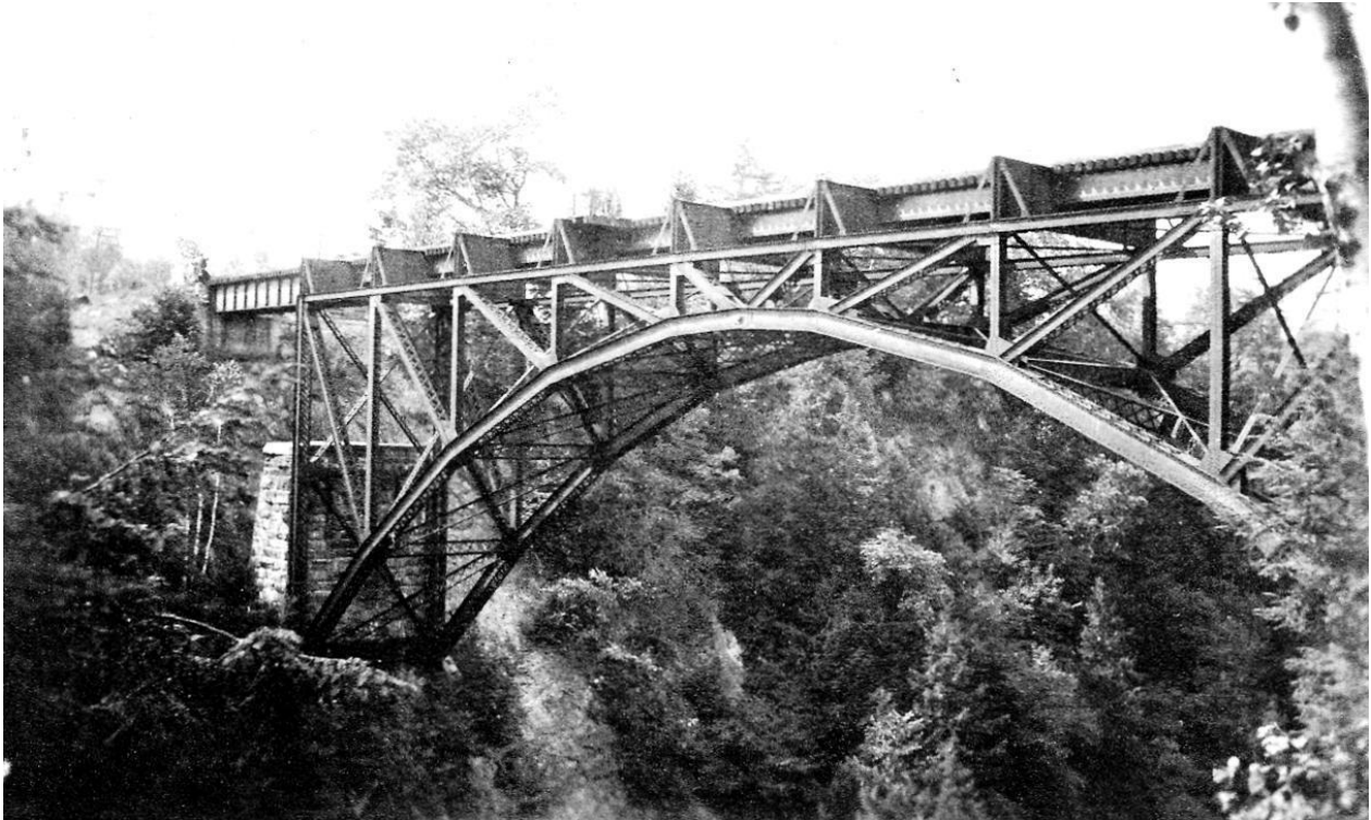
Figure 1. Quechee Gorge Bridge shortly after construction, in 1911.
